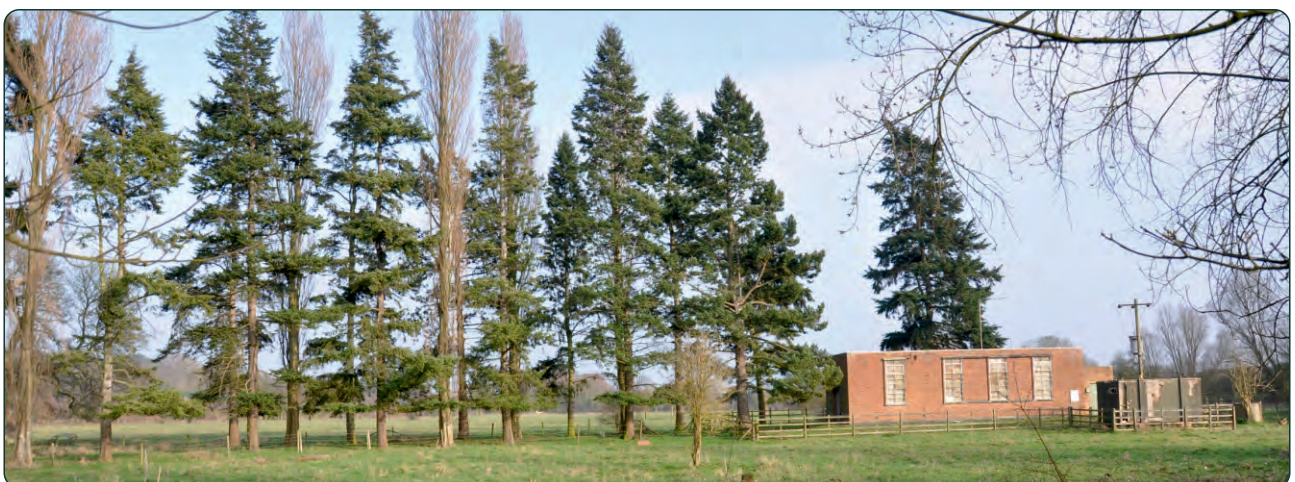
Photo F3. Eastern Pumping Station
